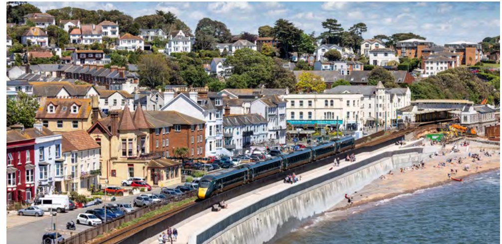
Specialist low carbon concrete was supplied for a new sea wall in Dawlish, Devon
