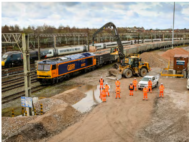
Hanson Aggregates Tuebrook rail depot opened in March 2021
